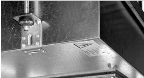
Figure 4 – "Z" suspensions
