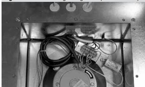
Figure 9 – Internal wiring arrangement (RPH series fan)
