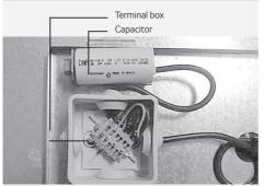
For single-phase fans a capacitor mounted outside the box terminals must be checked (Fig. 10).
