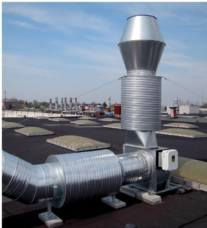
GEOVENT centrifugal fans LSFG/MSFG (with forward curved blades) and LEF/MEF (with backwards curved blades) are used for process extraction in industry or for comfort ventilation.
